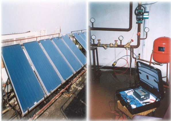
Solar system for hot water production installed in the old people's house in Silistra
